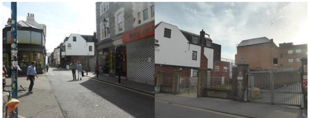
Figure 4: Gap in Ship Street streetscape from gates to Hippodrome & Dukes Lane
