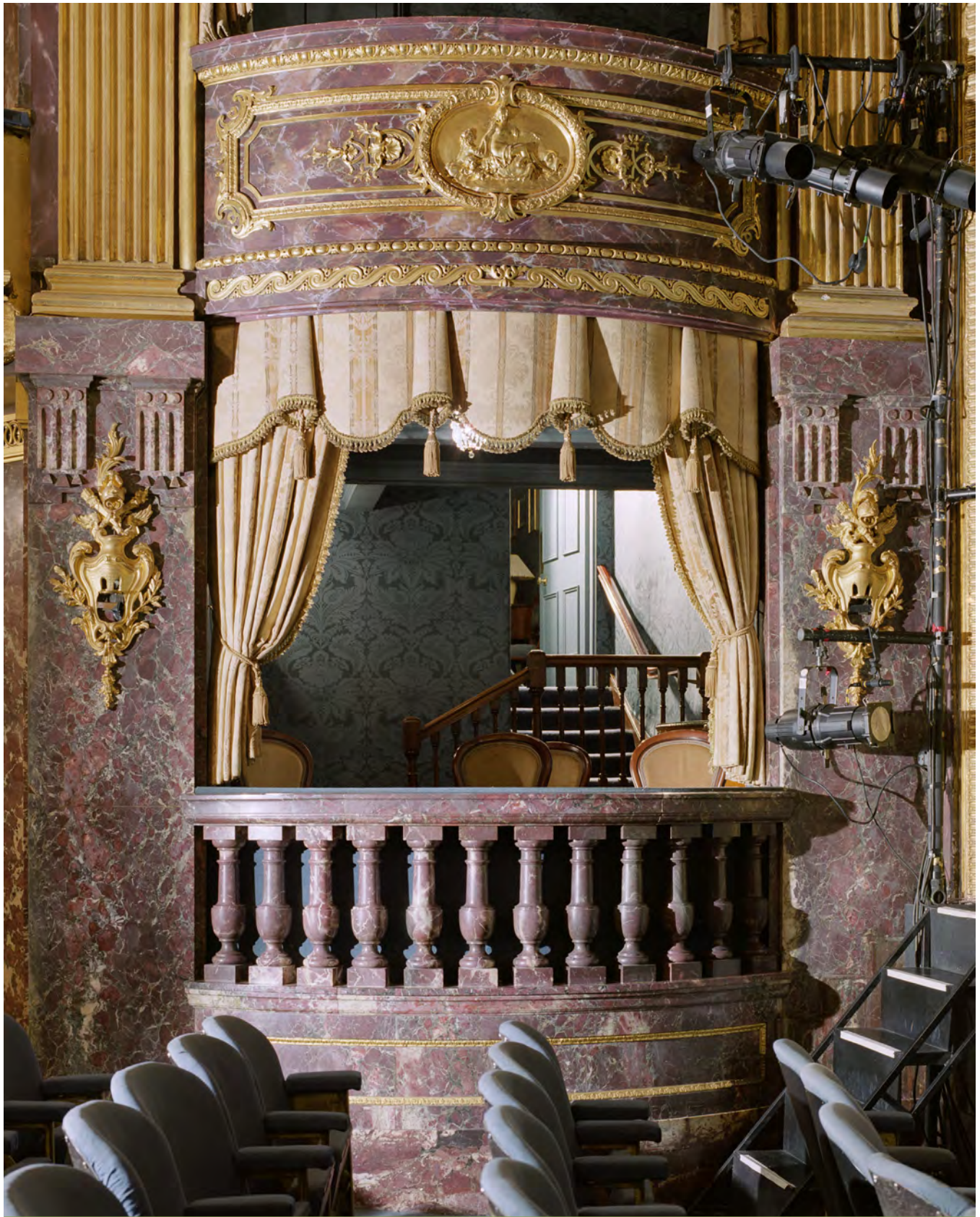
Figure 14: Haymarket Theatre, London (interior by Charles Stanley Peach, 1904). The illusion of sumptuous decoration is created by fibrous plaster, formed of simple materials.
