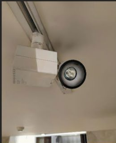
Existing Halogen lighting
