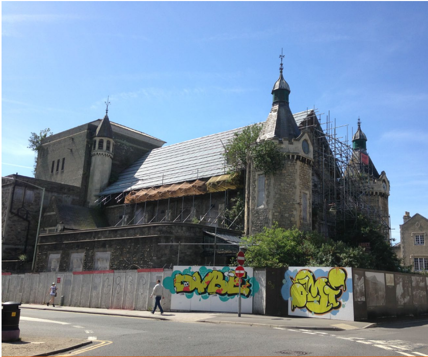
Swindon Mechanics' Institute
